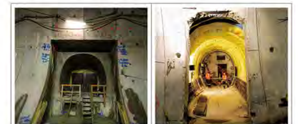
Cross Passage NATM Construction
